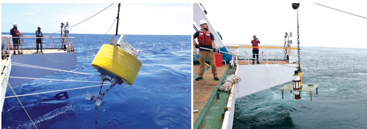
Deployment of SAIC Tsunami Buoy onboard Sagar Nidhi cruise in March 2020
